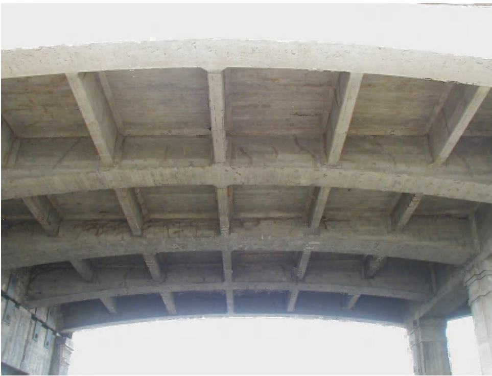
Figure 4: Typical view of girders and deck soffit.
