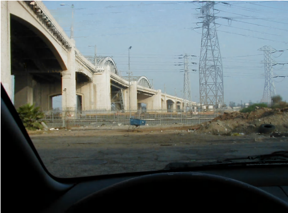
Figure 2: View of Sixth Street Viaduct looking east from approximately Bent 10.
