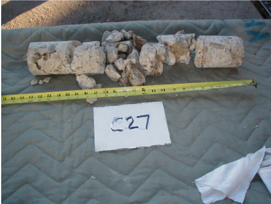
Figure 20: Internal cracking so severe that core broke into rubble during extraction.
