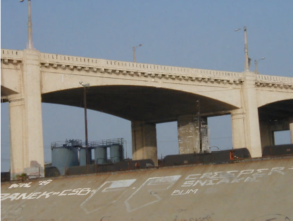
Figure 3: Span between Bents 12 and 13.
