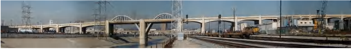
Figure 1: Overall view of Sixth Street Viaduct looking north between Bents 7 and 19.
