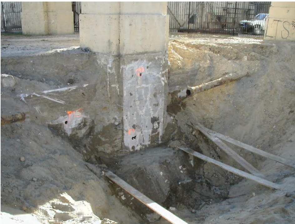
Figure 15: Excavation and core locations at Bent 23.
