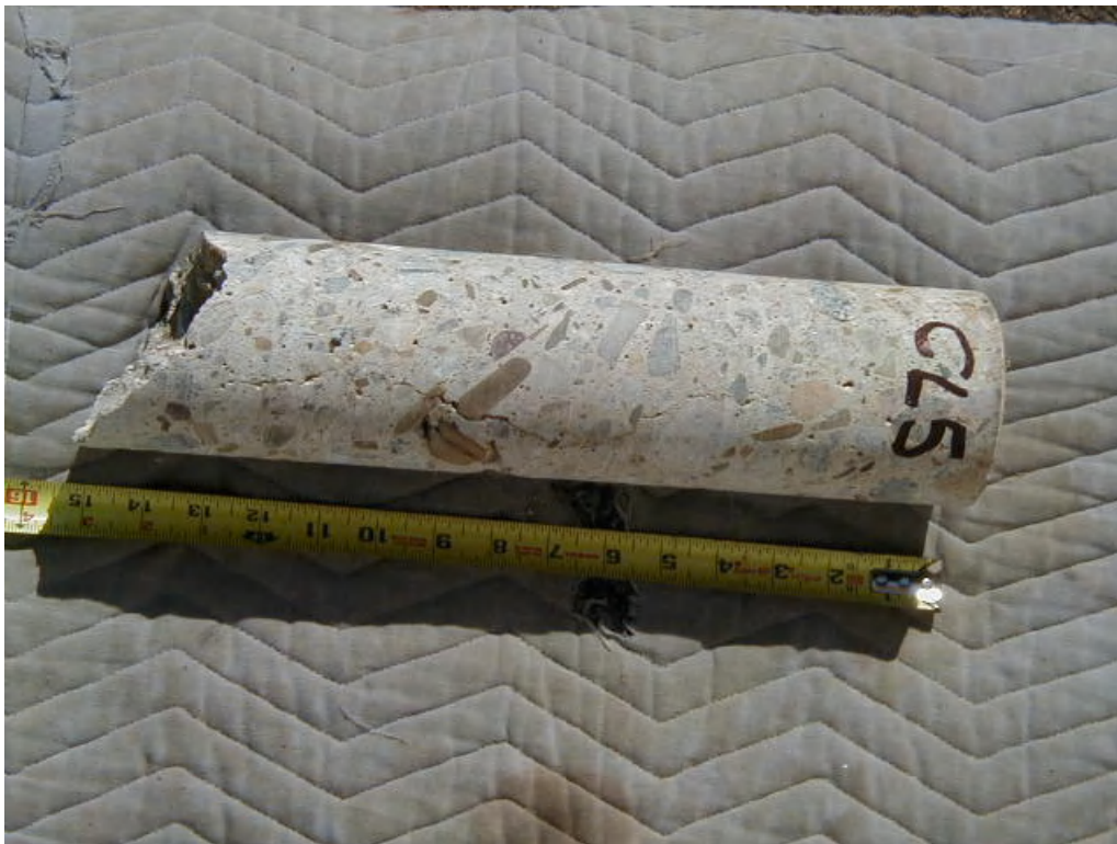
Figure 21: Example of a core with a moderate visual distress rating.
