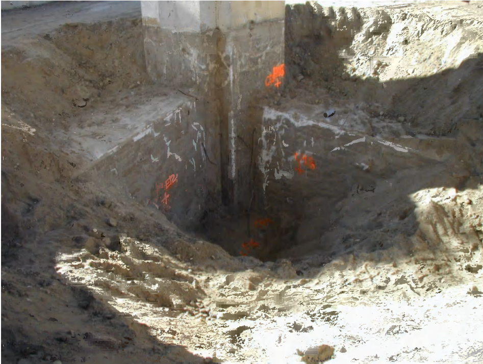
Figure 16: Excavation and core locations at Bent 21.
