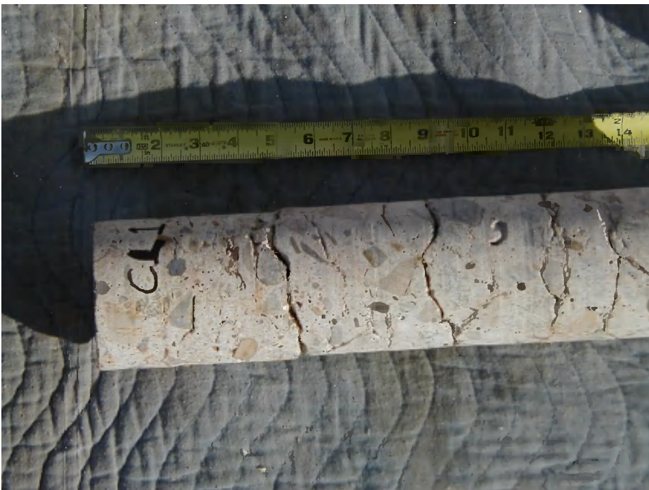
Figure 17: Typical pattern of network cracking seen in severely cracked cores.
