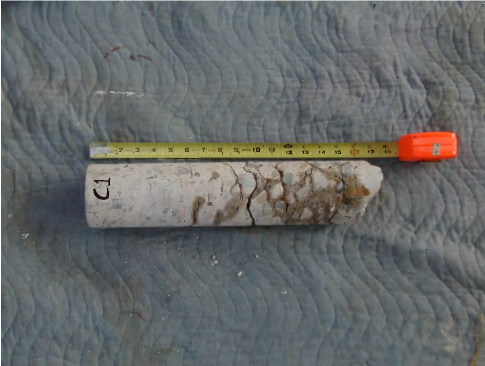
Figure 18: Network cracking was typically more severe deeper in the core than near the surface of the concrete.
