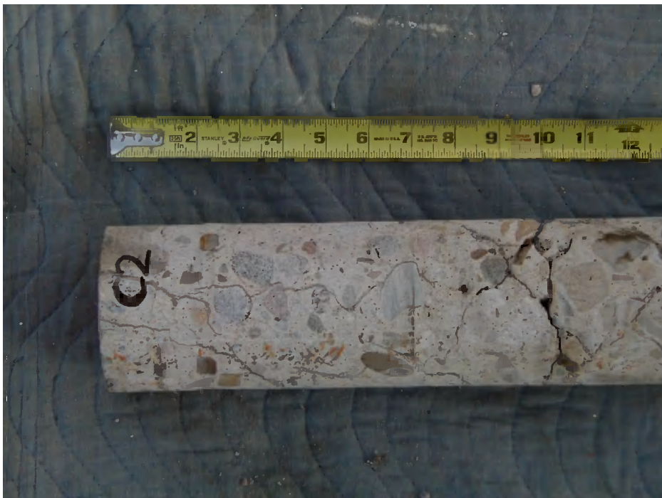
Figure 34: Close-up of portion of Core C2. Note the tested portion of the core had been previously injected with epoxy.
