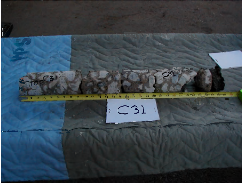
Figure 29: Severely distressed core with lowest f'_c = 1510 psi. Test made on portion from 1-inch to 7-inch depth. Core 31, girder diaphragm above bent cap at Bent 9.
