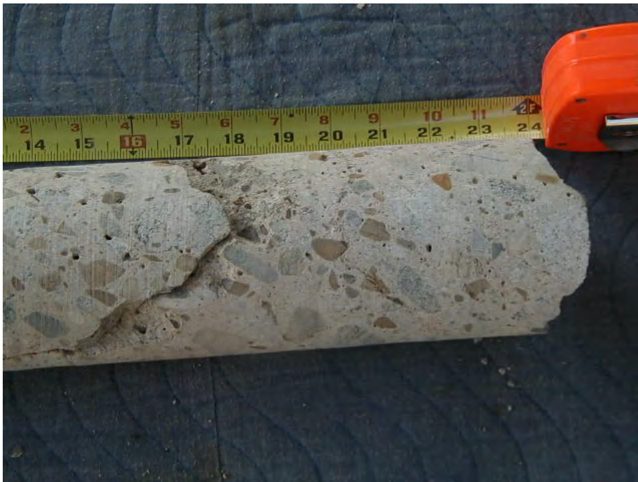
Figure 37: Close-up of portion of Core C6 that was tested.
