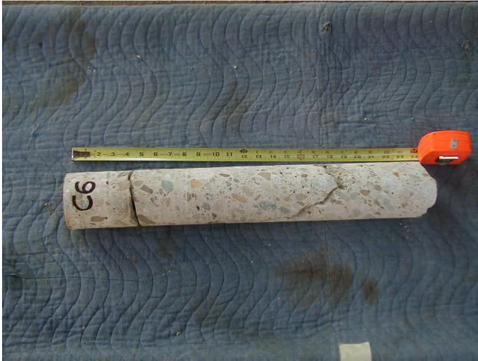
Figure 36: Core with medium distress that had highest compressive strength value of all cores, f'_c = 5770 psi. Test made on portion from 19 ½-inch to 23 ½-inch depth. Core C6 from south column, east elevation at Bent 33. Total column thickness is roughly 9 feet.
