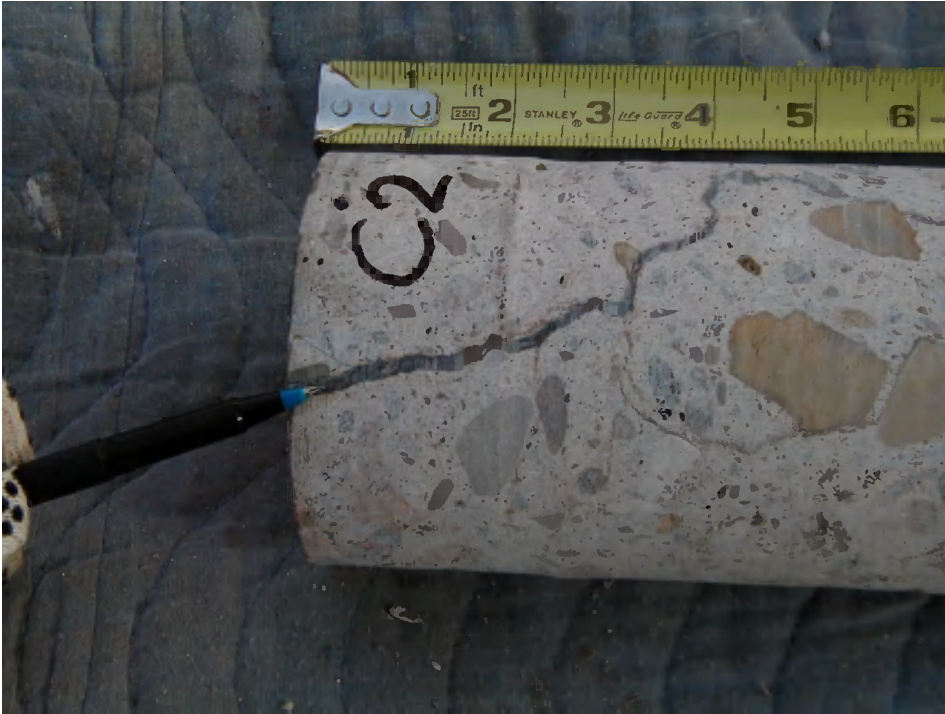
Figure 28: Core with a portion of an epoxy injected crack. Note that the fine cracks have not had penetration.
