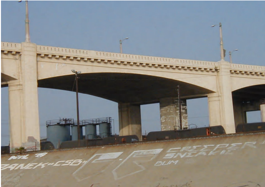
Figure F.5. Span between Bents 12 and 13
