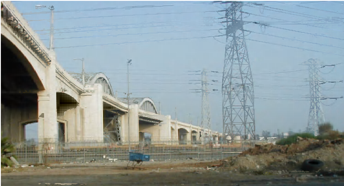
Figure F.2. View of the Sixth Street Viaduct looking east from approximately Bent 10
