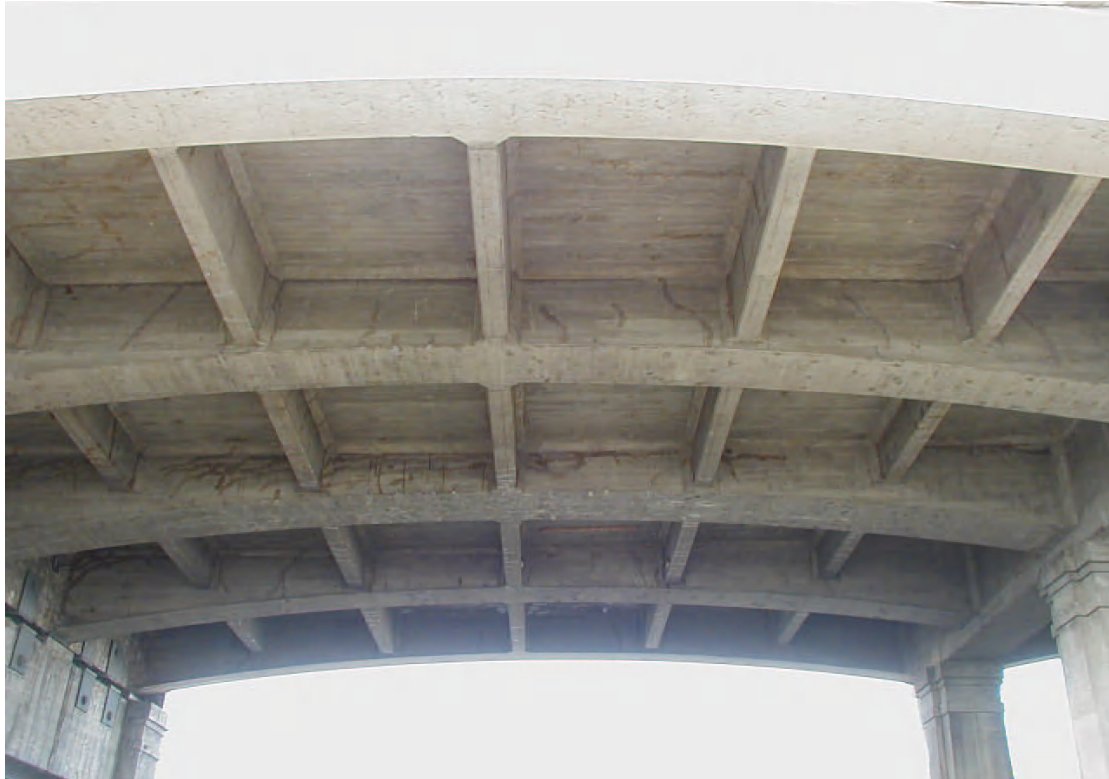
Figure F.6. Typical view of girders and deck soffit
